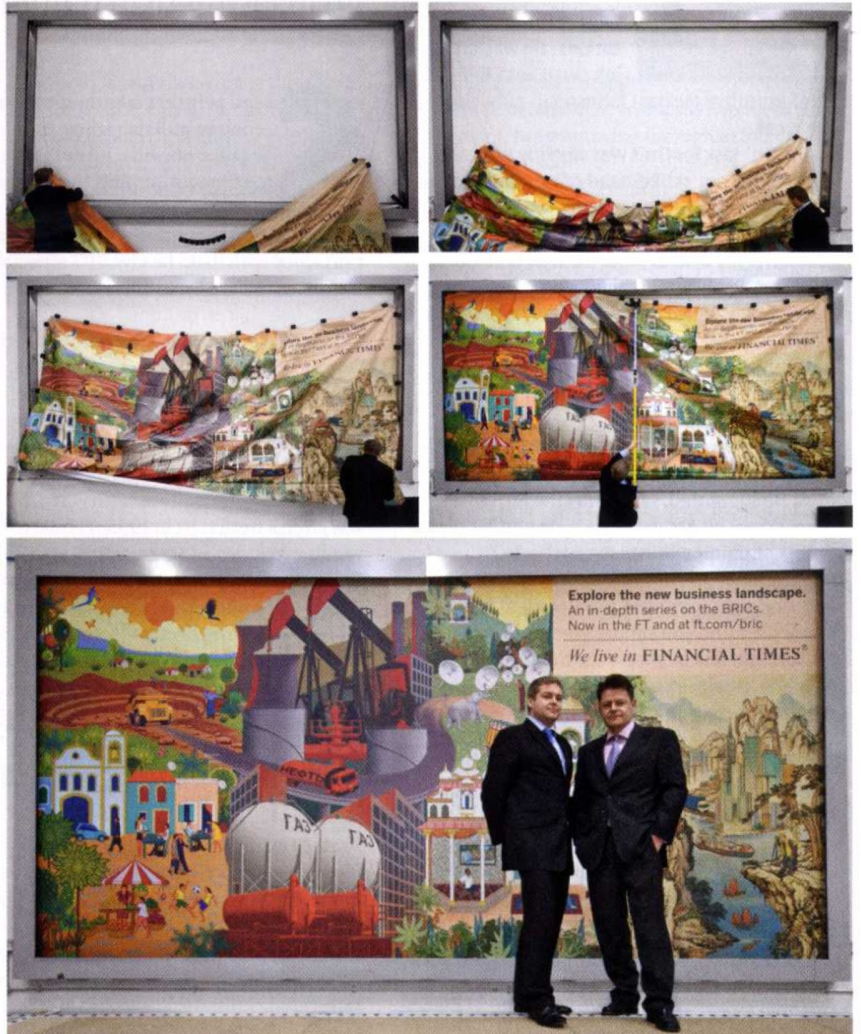
Ecoflex is a polyethylene-based outdoor poster system that does away with messy paste-ups
